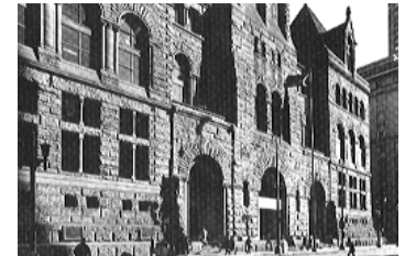
Allegheny County Courthouse
